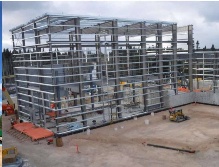
Continued construction on copper flotation area, late October 2020
