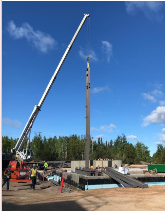
First beam installed on flotation building, early September 2020
