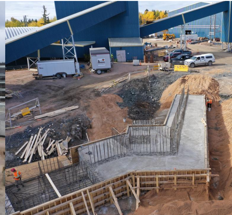
Haul ramp for ore receiving, late September 2020
