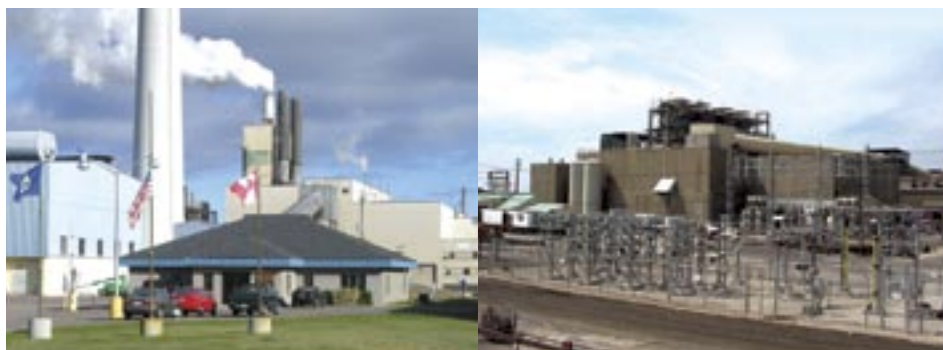
(Left) The White Pine Copper Refinery in Michigan. (Right) The zinc plant's state of the art electrolytic cellhouse in Flin Flon.
