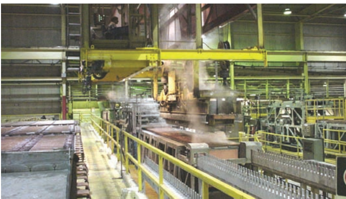
Crane and cathode stripping machine at White Pine Copper Refinery cellhouse
