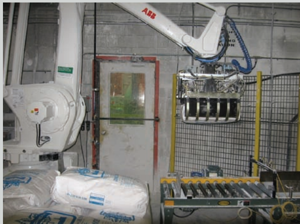
One of two robots installed at Zochem
