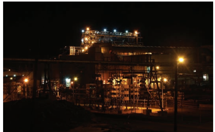
Zinc cellhouse at Flin Flon
