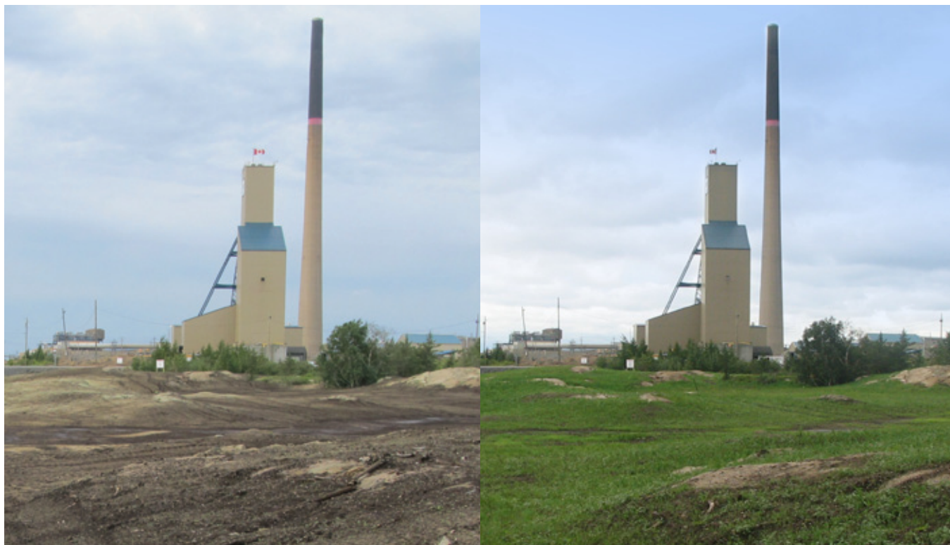
↑ Hydroseeding depicted at Mouse Pond, north of the 777 mine (before visible growth) and hydroseeding depicted at Mouse Pond after visible growth.
