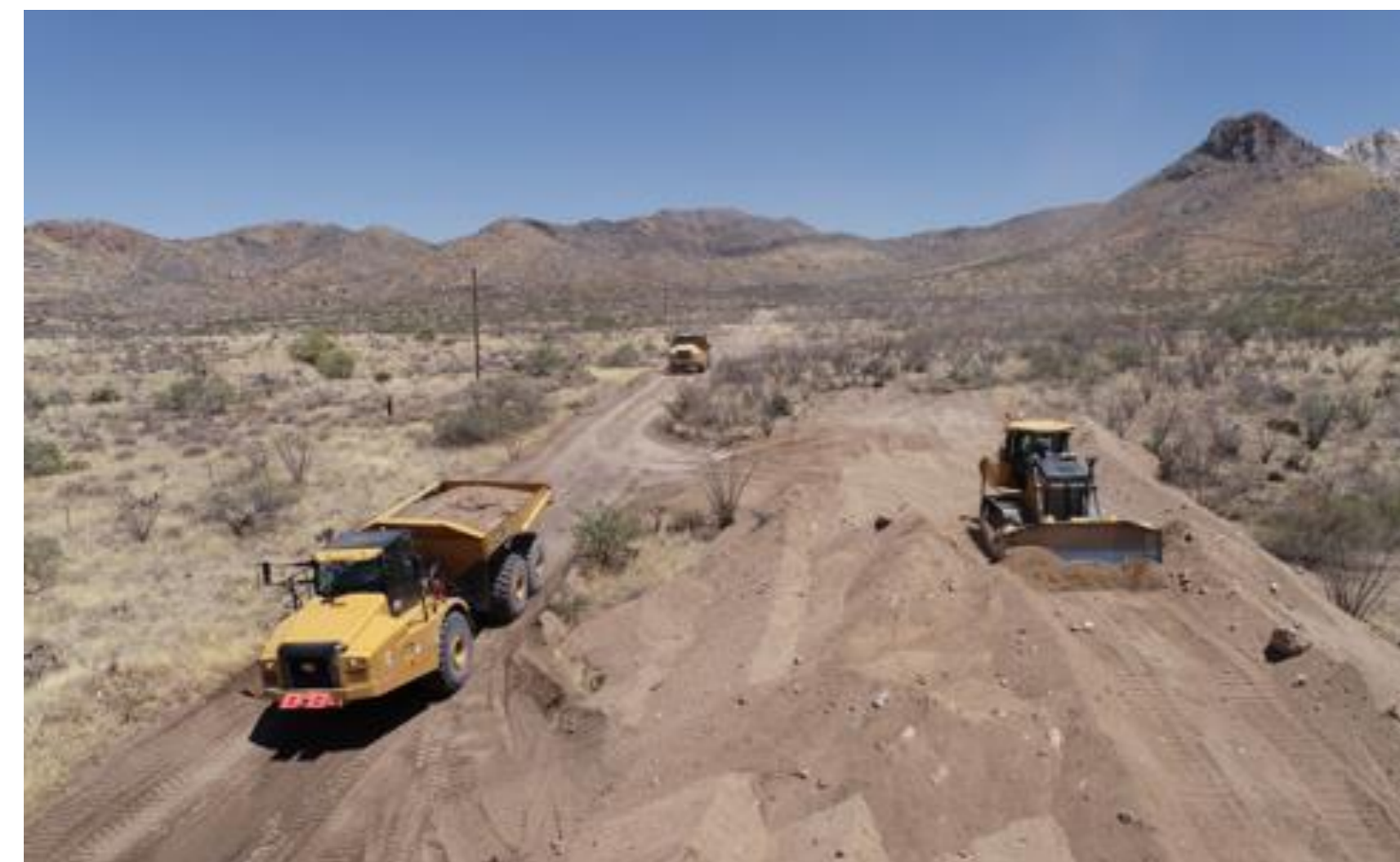
Phase I land clearing in proposed tailings areas, May 2022
