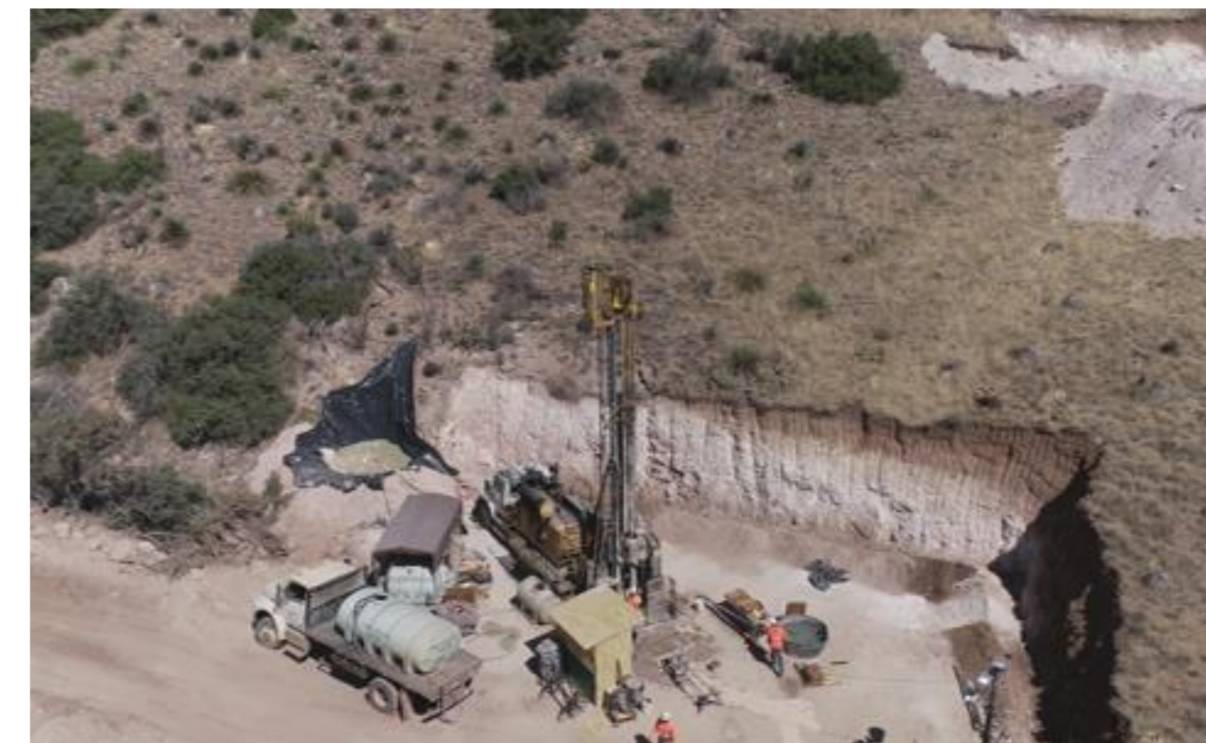
Drill rig at Bolsa deposit, May 2022
