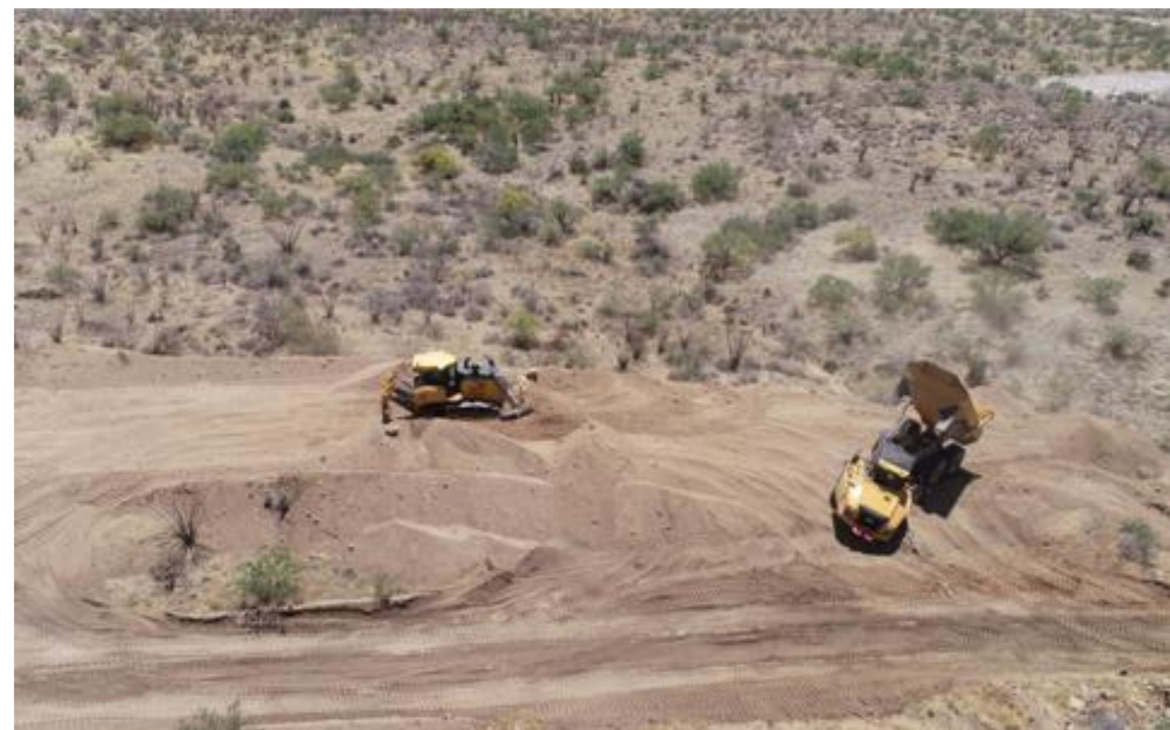
Phase I land clearing in proposed tailings areas, May 2022
