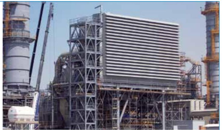
Our large air filtration systems help protect our Customer's gas turbines and help meet the growing global demand for electricity
