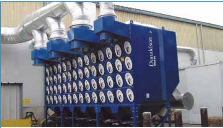
Our Donaldson® Torit® Downflo® Oval Dust Collector at a titanium grinding operation
