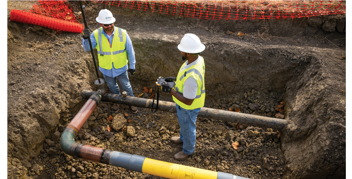
Gas techs installing new pipe for a relocation project.
