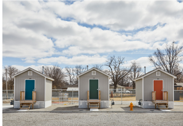
Simulation City at the ONE Gas Training Center allows employees to gain hands-on experience locating utilities, identifying simulated leaks and addressing code violations.
