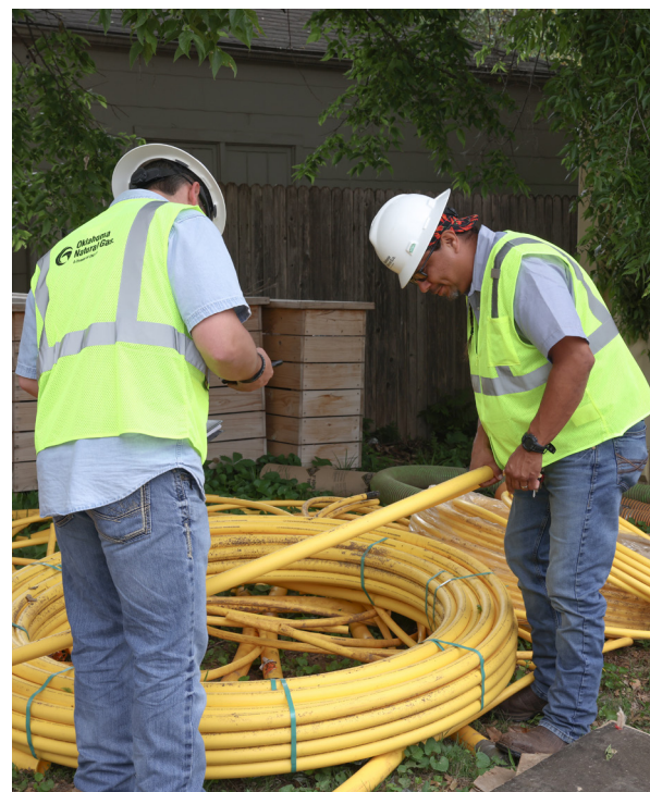
Field inspectors using the material tracking application.
