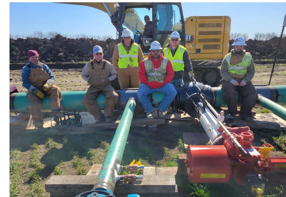
Kansas Gas Service team members pose for a photo while replacing a transmission line in Cunningham, Kansas.
