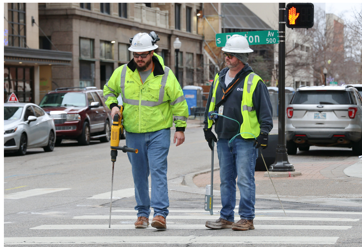
A leak survey team inspects natural gas lines in downtown Tulsa, Oklahoma.
