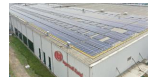
Main Workshop Roof
