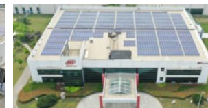
Office Building Roof
